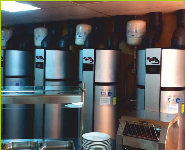
Example of piggy backing units for commercial capacity
